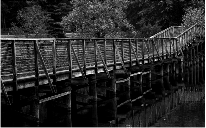
Bridge at Smallwood State Park, by Paul Toscano
